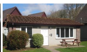
Bungalow No 91 at Hengar Manor
